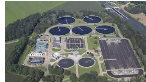
4. Maintenance and installation of equipment in sewage treatment plants
