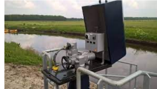
2. Mechanical and electrical works
