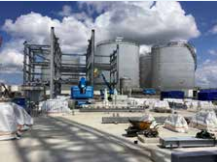
Structural Steel Erection Process Building
