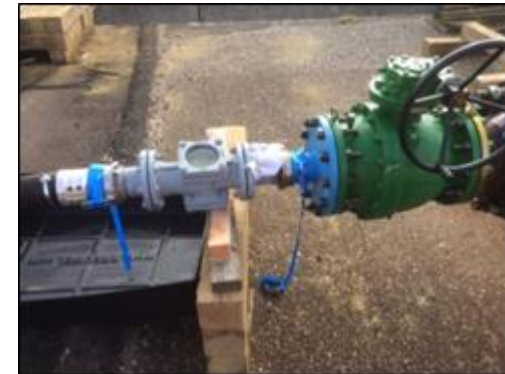
Outlet of the pipeline
