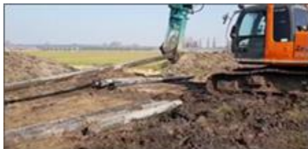
NEAR SHORE PULL & CUT
